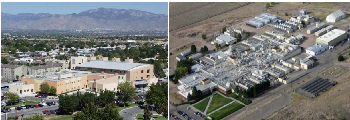
North and South facilities for Lovelace Respiratory Research Institute in Albuquerque, NM comprising 125,000 and >350,000 ft 2 of research space.
